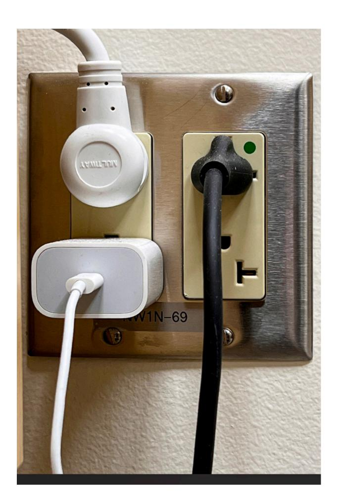
The equipment grounding wire is connected to the grounding prong at the receptacle outlet, which is connected to an equipment grounding wire in the branch circuit wiring back to the main electrical panel.
